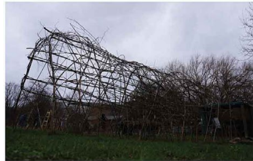
Test 1: Community workshop for 1:1 living willow tunnel
