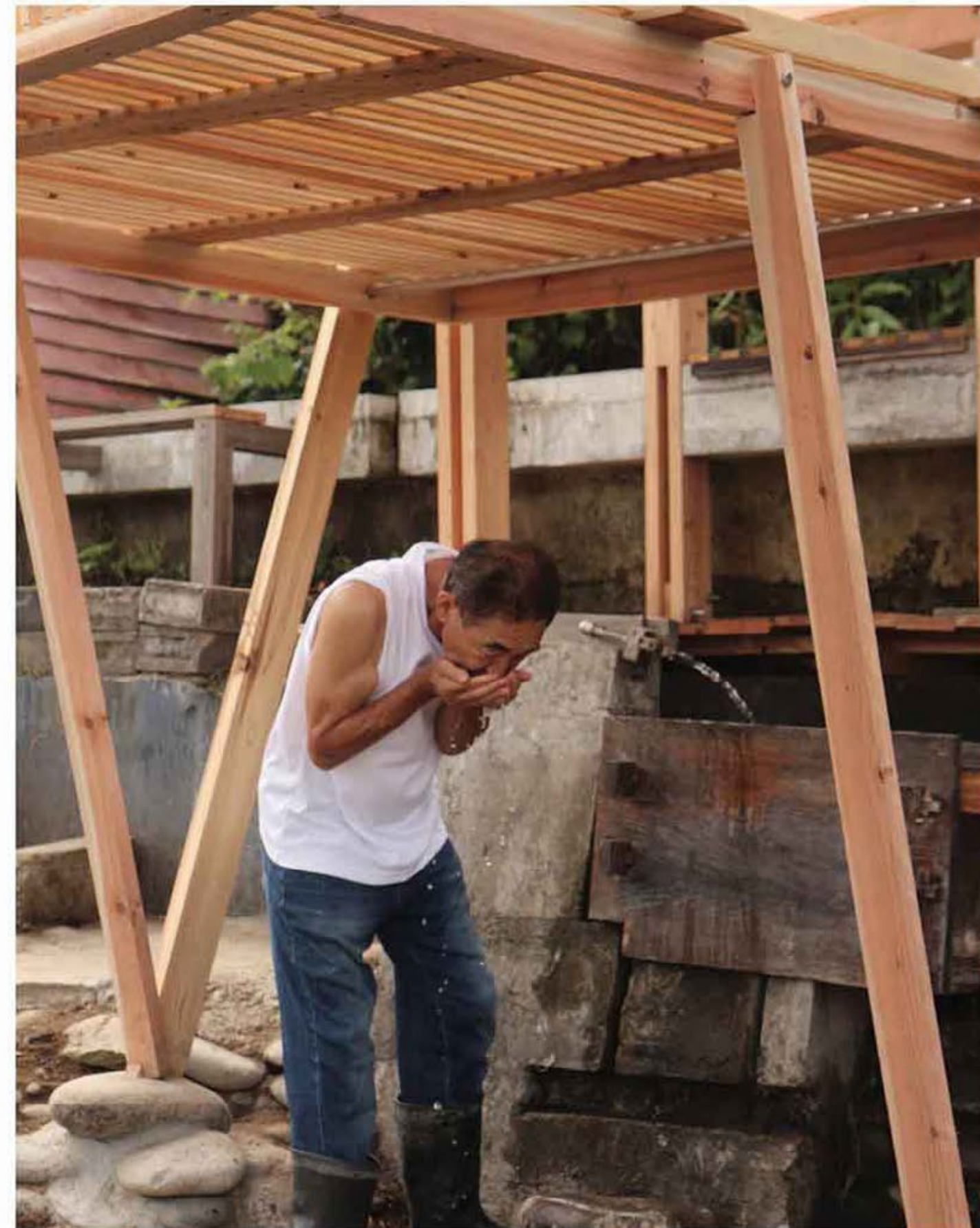
A local villager and friend named Hirosun, enjoying the fresh spring water after repair of water channel upon project completion
