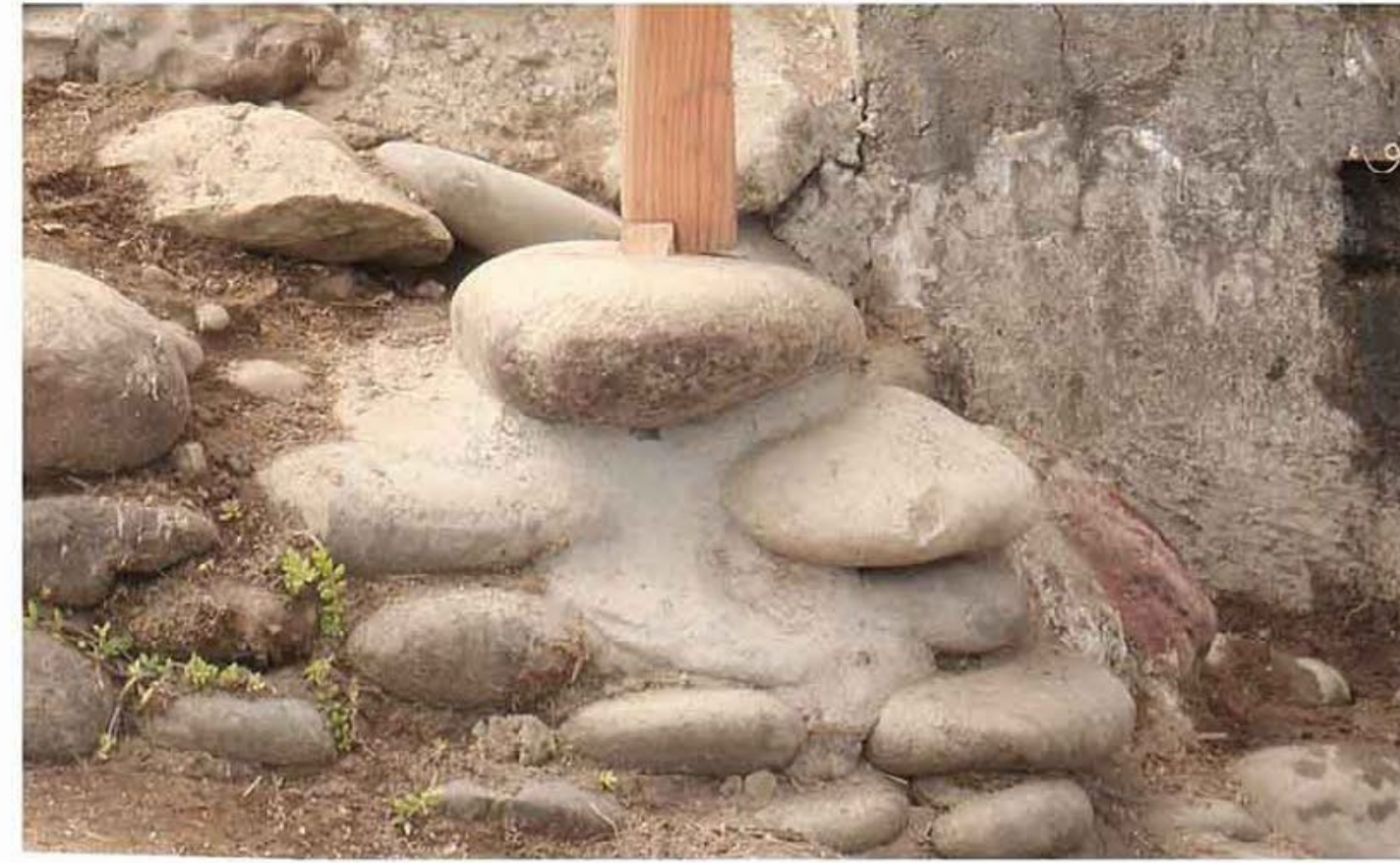
Dry-stacked stone and concrete-stabilised base, supporting timber post
