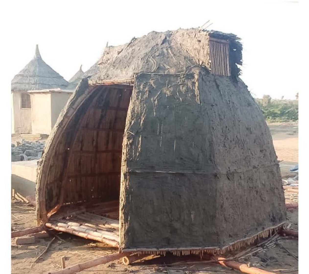
Bamboo pod clad with a thin layer of earth-lime plaster to provide shelter
