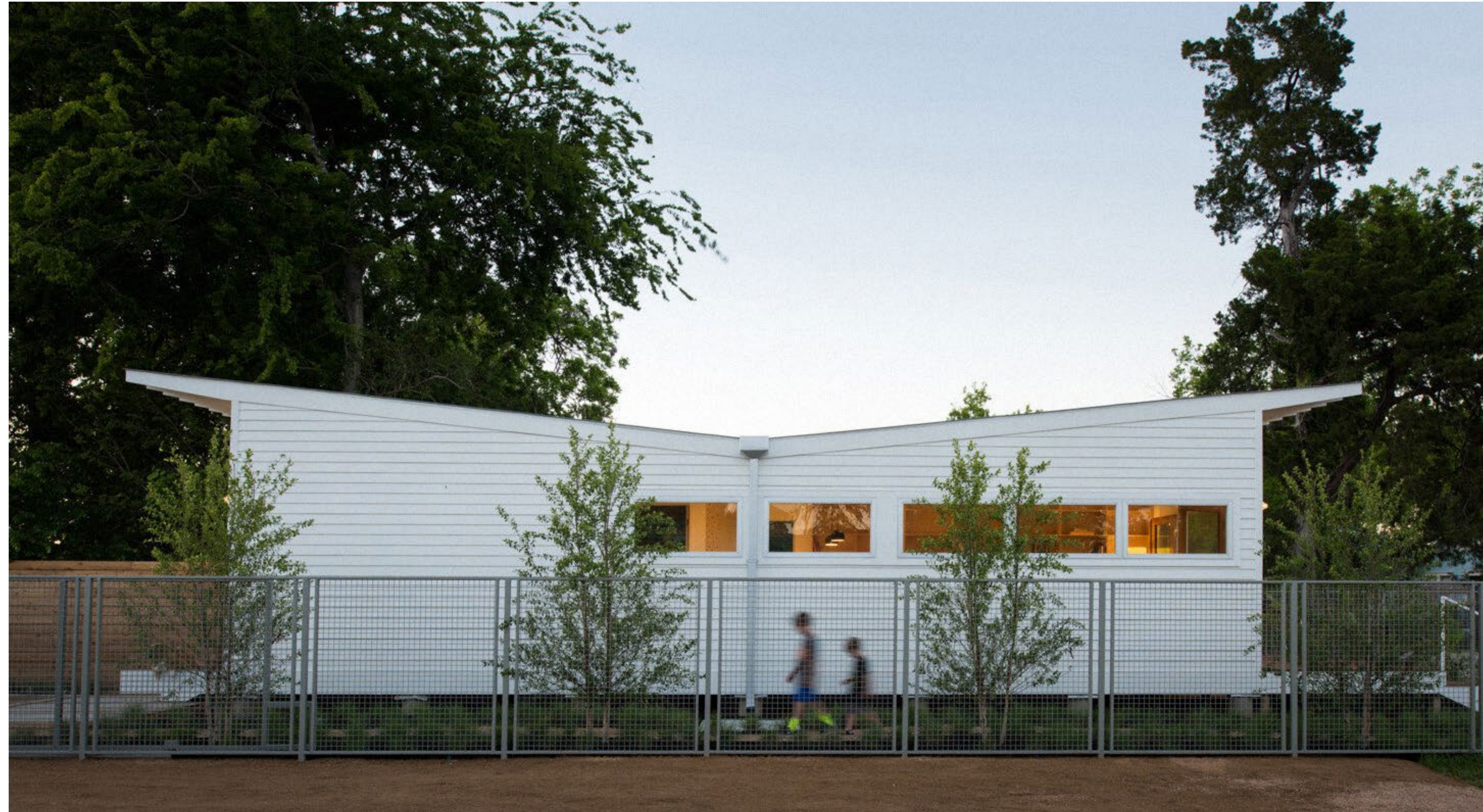
Image of the built zFAB, a typology for which I produced the drawing set during my work experience, under the supervision of the managing architectural designer. Image is property of Brett Zamore Design.
