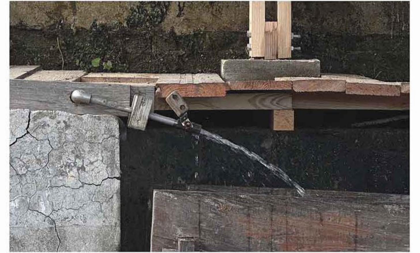
Wood and metal water spout system, to provide adjustable pressure of fresh water stream
