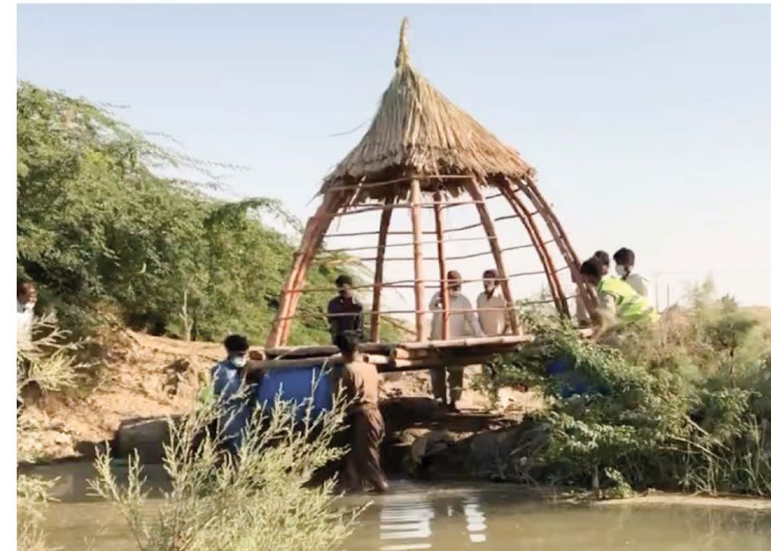
Bamboo pod covered with thatch roof to test lightweight roofing system before testing structural buoyancy
