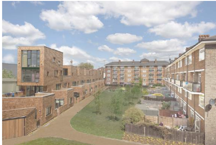
Figure 2.1: Hannibal Road Gardens before paving (2011)
