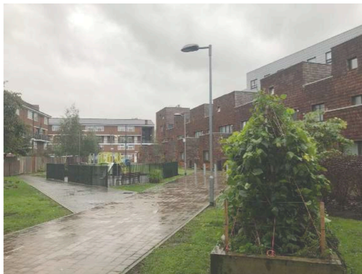
Figure 2.2: Hannibal Road Gardens Courtyard after paving (2019)
