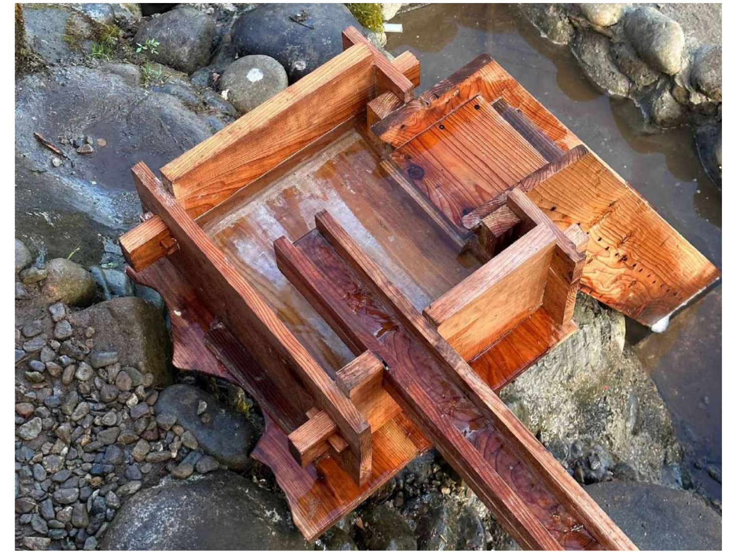
Timber sink with a wooden water channel directing fresh water stream into designed concrete-cast pebble basin.
