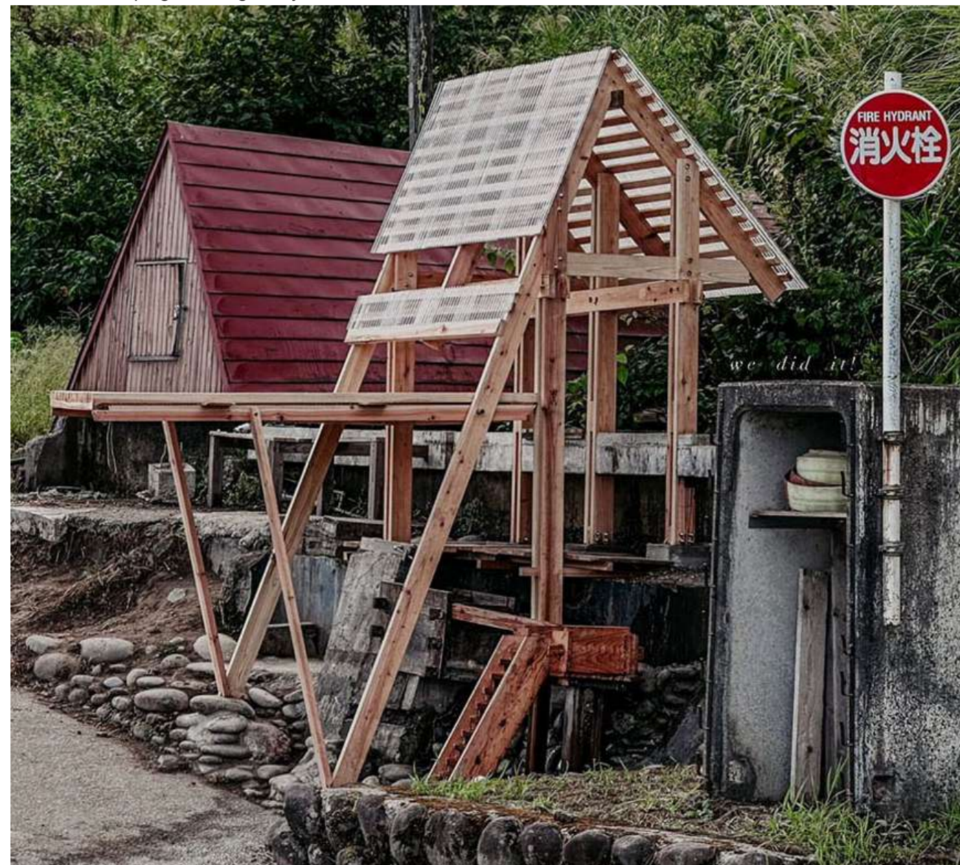
Completion of Watermelon Place project, July, 2023
