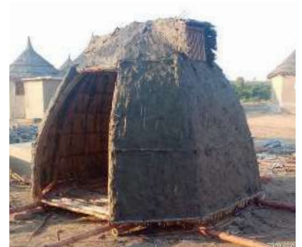
Bamboo Pod clad with thin layer of earth-lime plaster to provide shelter
