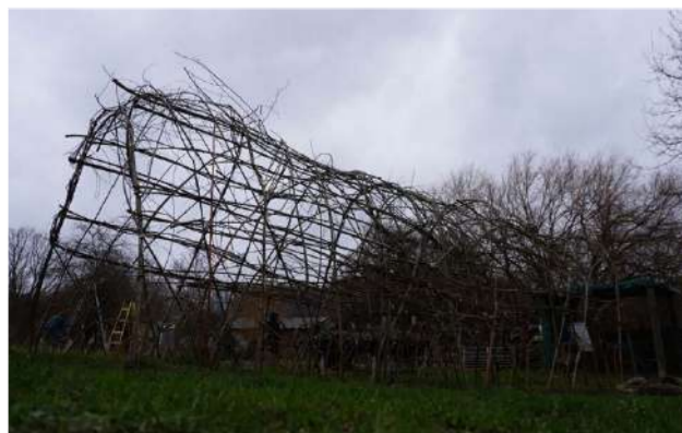
Test 1: Community workshop for living willow tunnel
