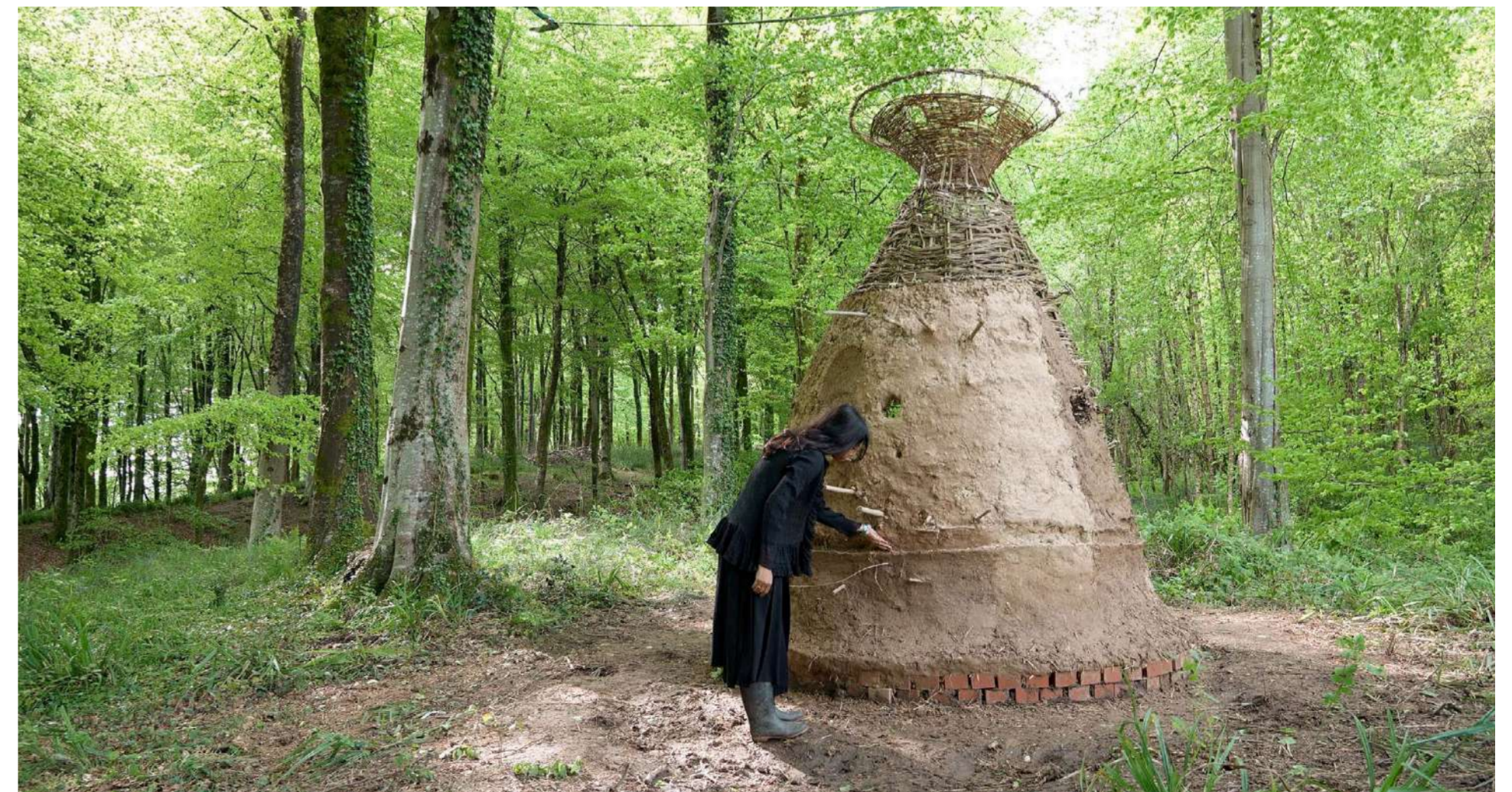
Meticulously woven NEST structure, built in Hooke Park, Dorset, UK using regionally sourced willow and cob
