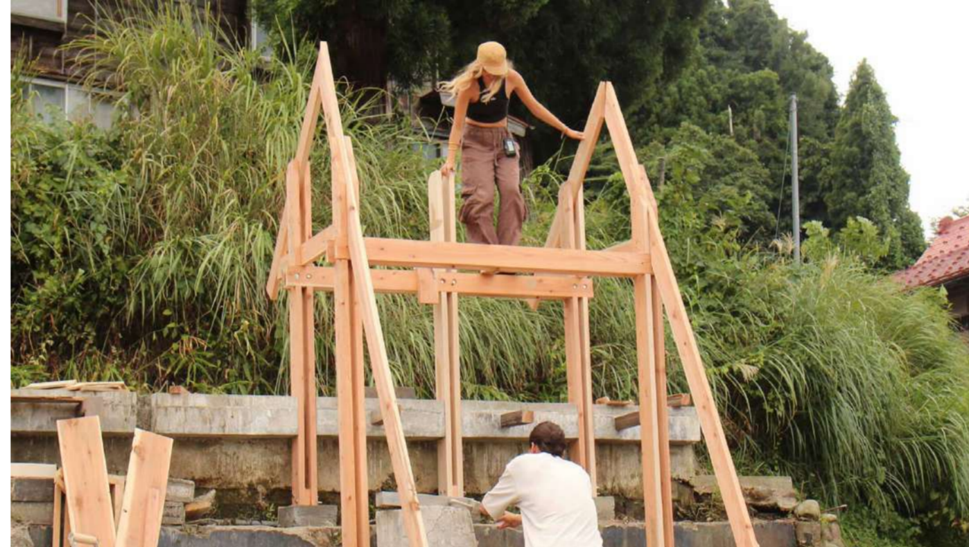
Construction in progress using locally sourced timber
