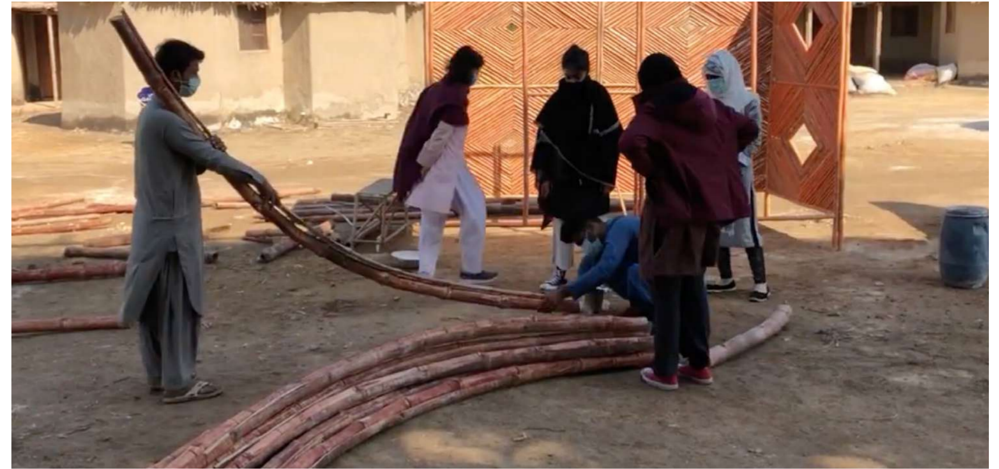
Using scoring method to bend dried bamboo
