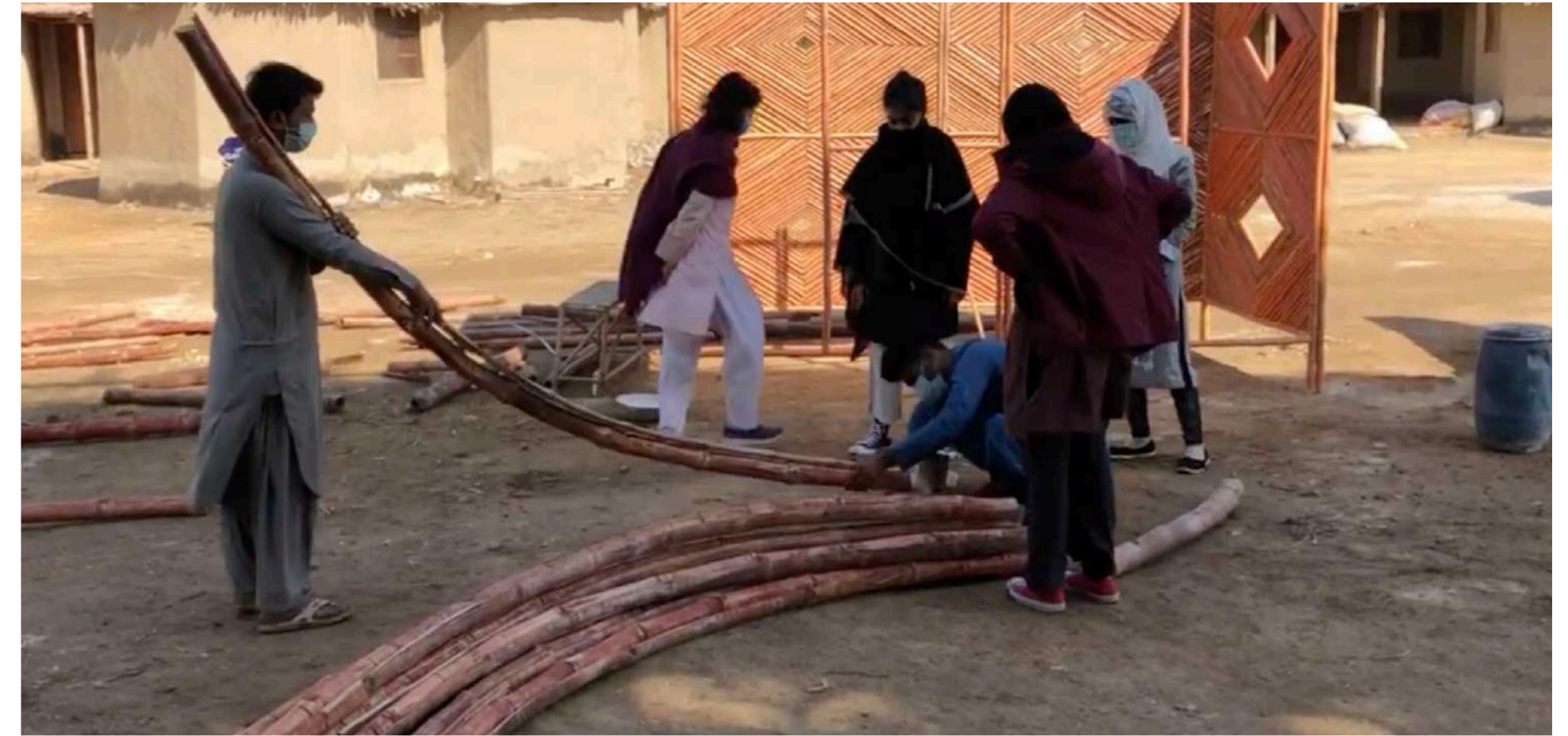
Using scoring method to bend dried bamboo
