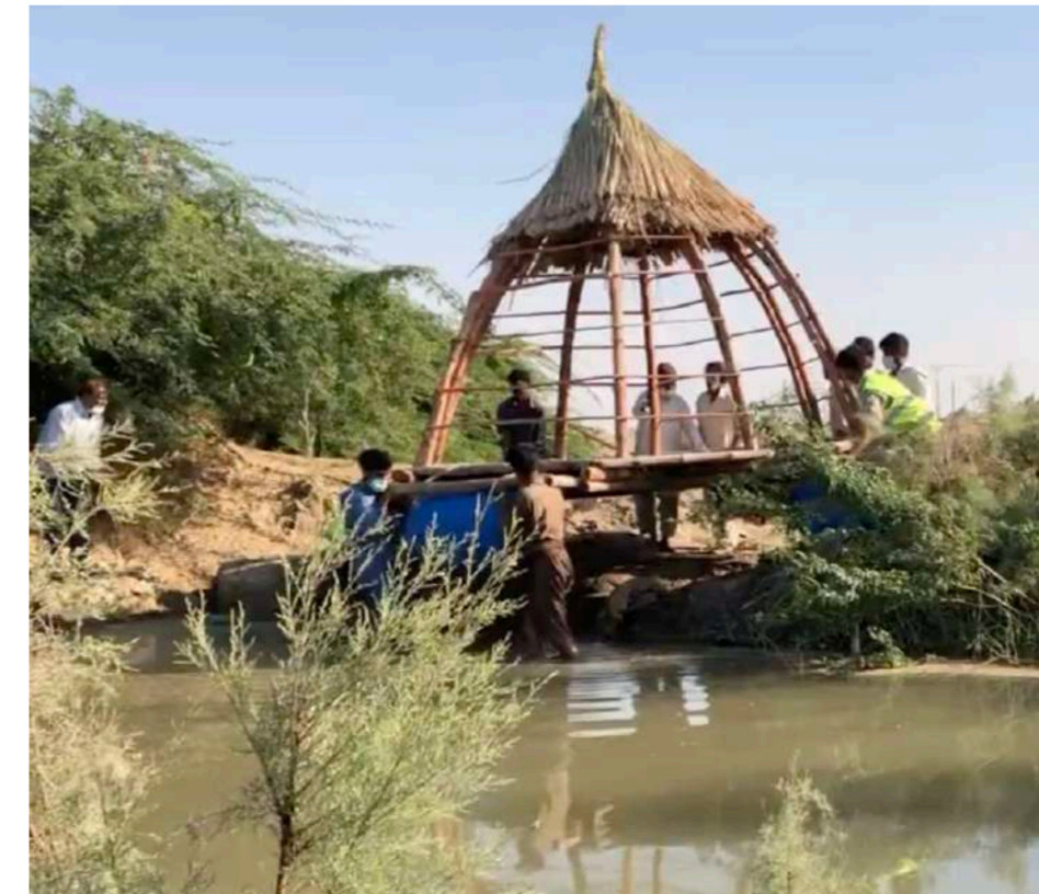
Bamboo pod covered with thatch roof to provide shade before submerging into canal
