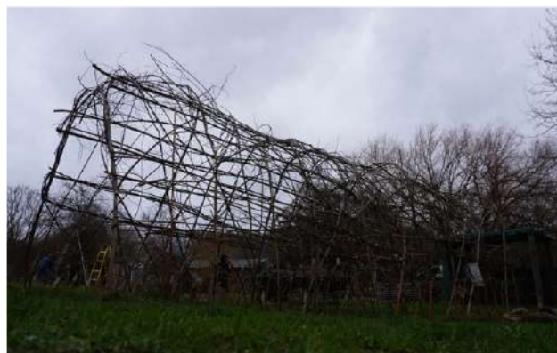
Test 1: Community workshop for living willow tunnel
