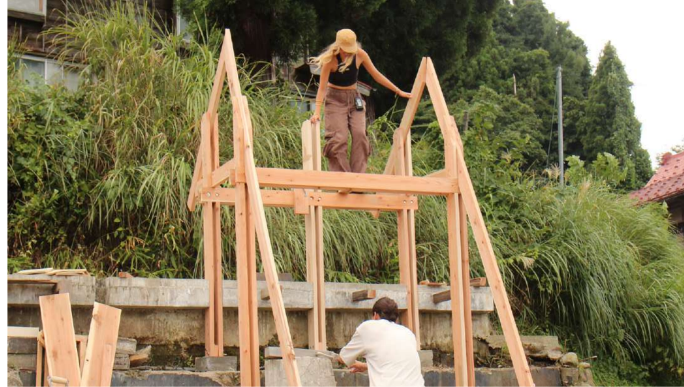
Construction in progress using locally sourced timber
