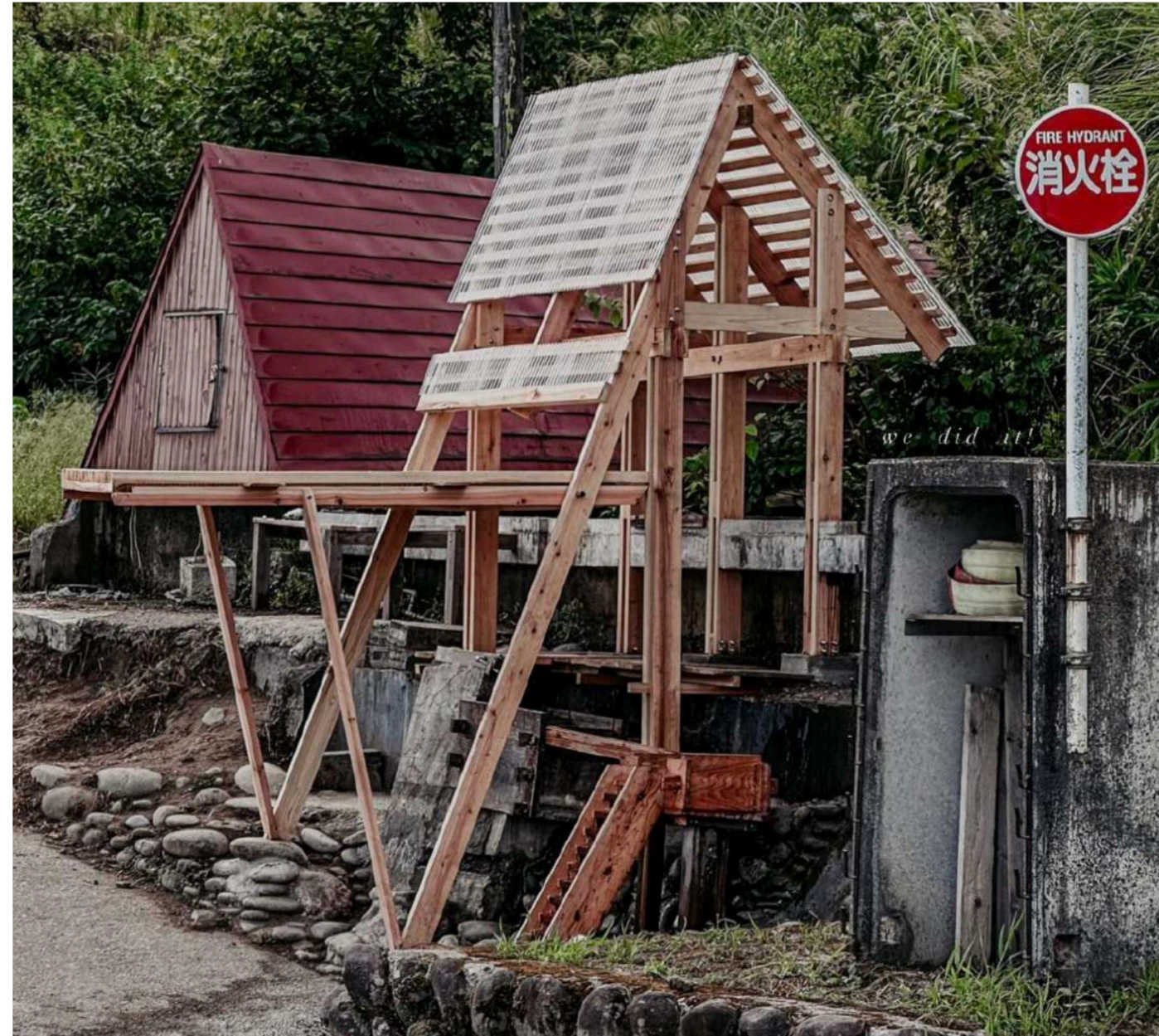
Completion of Watermelon Place project, 2023 July
